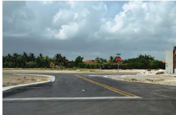
SW 136 St and Onsite Roads Completed Up to the First Lift of Asphalt and Temporary Pavement Markings
