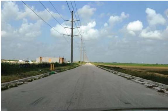
SW 136 St and Onsite Roads Completed Up to the First Lift of Asphalt and Temporary Pavement Markings
